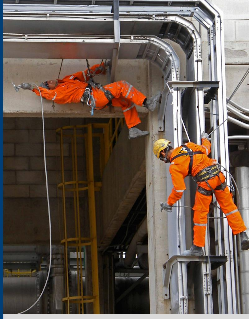
Fire Security's coating applicators employing rope access techniques to ensure total coverage for our clients turnkey cable maintenance operations.
