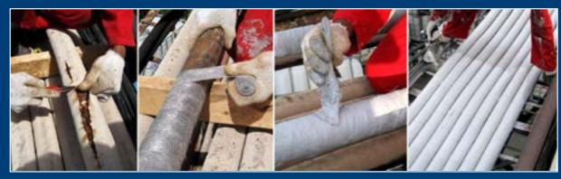
FS coating system for cable repair, lifetime extension, and fire protection can save millions compared to replacing old cables, here from a project at an industrial plant.
