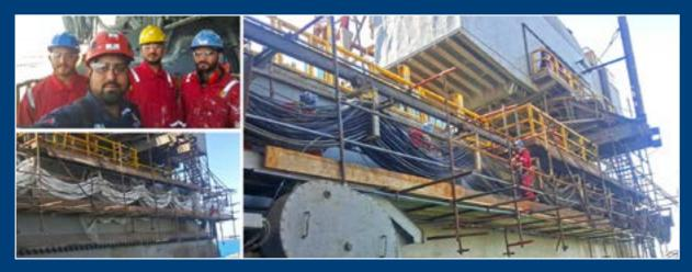
Our cable coating system is unique: it can repair damaged cables and offer fire protection in one operation. Failing to repair damaged cables can leave your rig, vessel, or industrial plant severely impaired.
