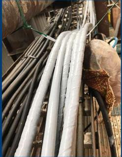
Oil, drilling mud and hydraulic fluid softens and damages cable sheaths. FS repair system is resistant to this hydrocarbon degradation, ensuring our cable repair will extend the life of cables exposed to the harshest conditions.
