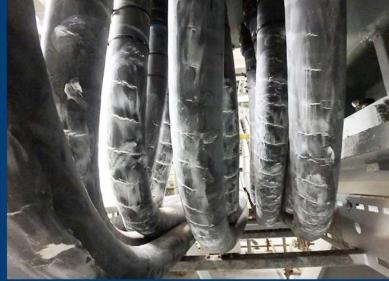
FS coating is applied to encapsulate the cables. The coating will restore any loss of the cables electrical integrity and upgrade the cables fire technically accordingly with IEC-60331 standard. Our coating is highly elastic and will cope with any minor movement in the cable outer sheath.
