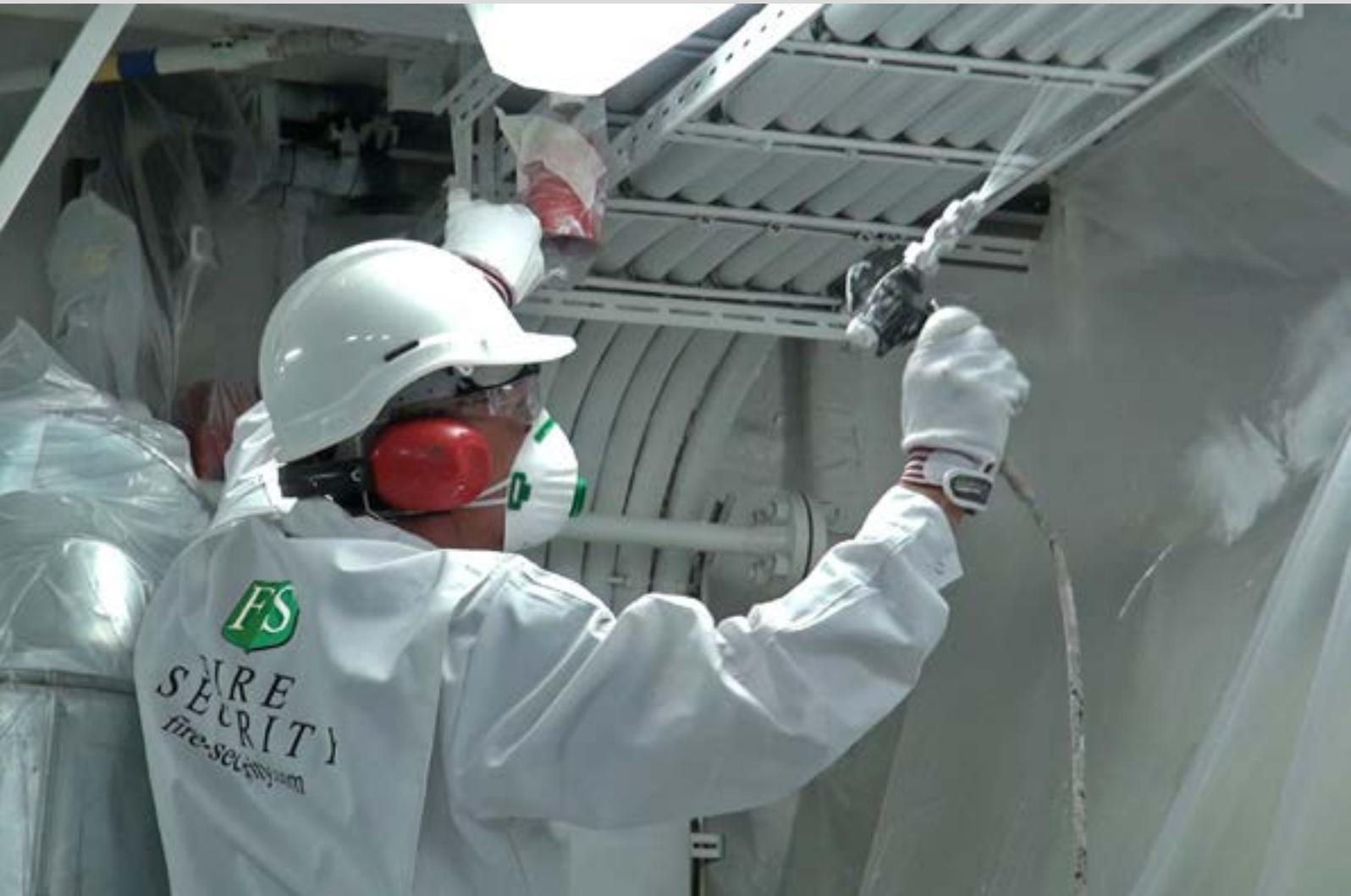
*Water Based Ablative FM Approved Cable Coating for the fire protection of electrical cables up to 90 minutes.*
