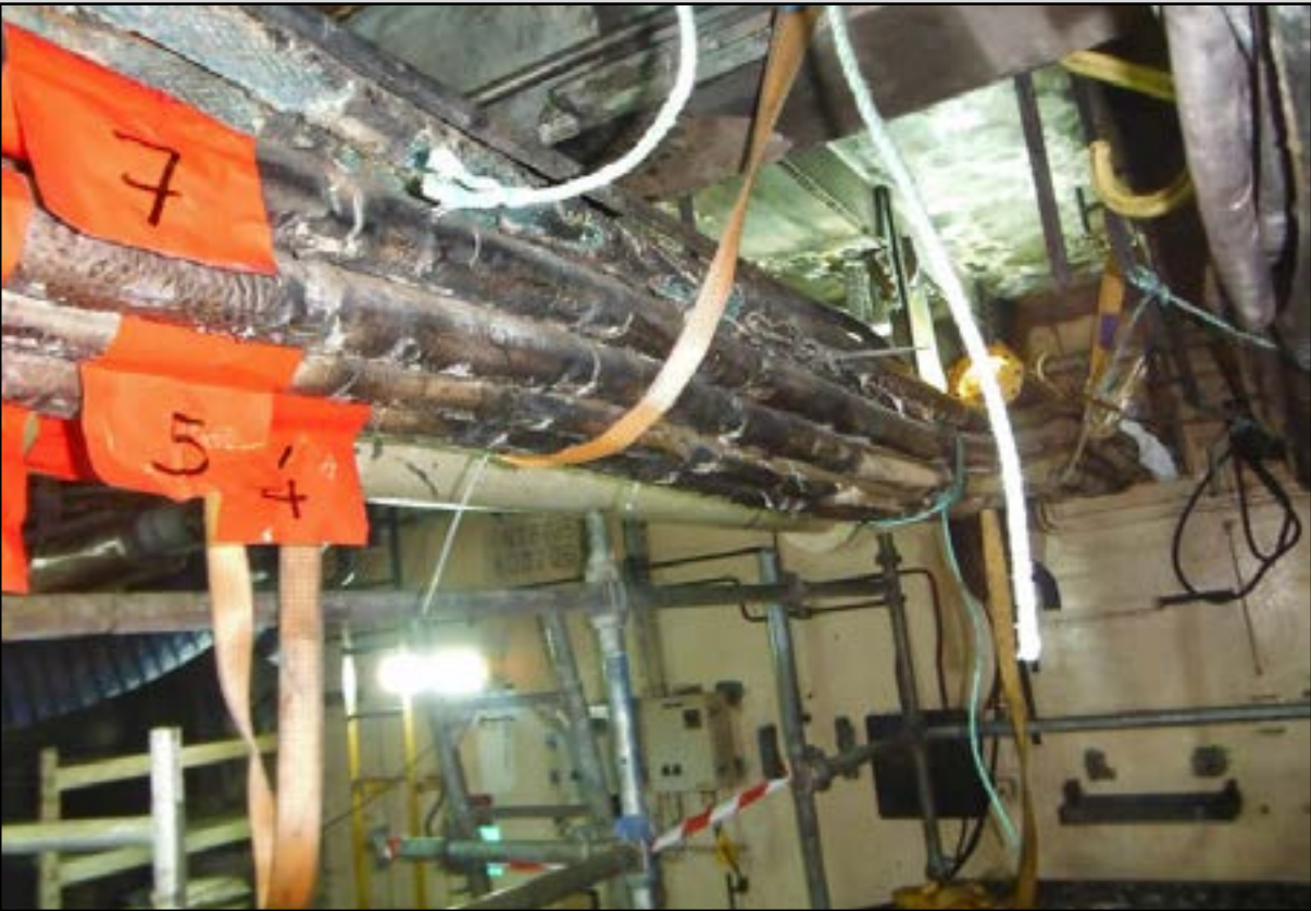
Cables that have been affected by fire but are still capable of operation. FS17 tape repair and coating with FS5.
