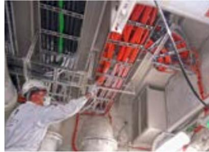
During a fire, the coating expands and protects the cables from fire damage and also prevents the fire from spreading via the cable trays. FS coated cables function during a fire, and if the fire is ceased within a reasonable time, there will be no need for cable replacement.
