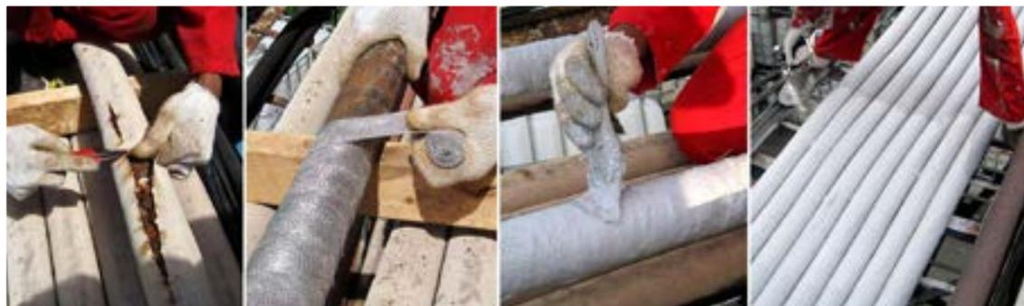
FS coating system for cable repair, lifetime extension, and fire protection can save millions compared to replacing old cables, here from a project at an industrial plant.
