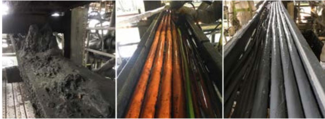
Our cable coating system is unique: it can repair damaged cables and offer fire protection in one operation. Failing to repair damaged cables can leave your industrial plant severely impaired.
