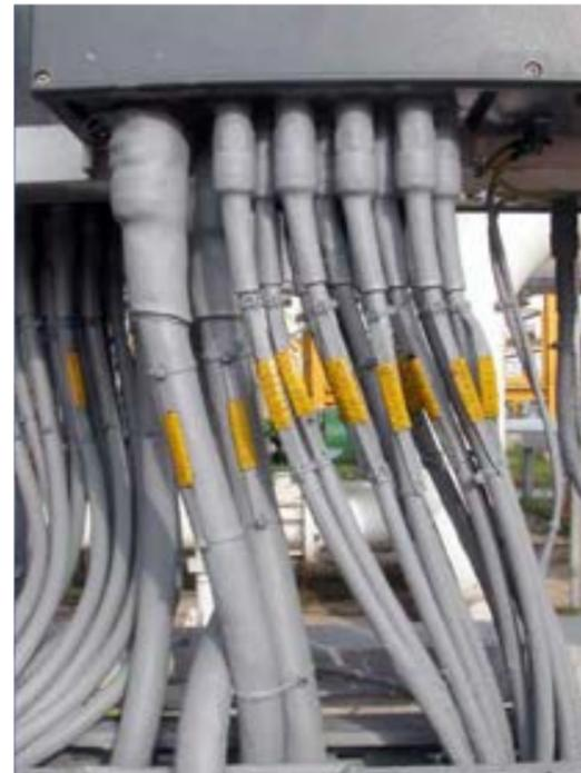
Fire Security's Class approved coating systems are perfect for repairs and environmental protection in high-risk areas in both offshore and land-based industries and lately on numerous LNG carriers and refineries.
