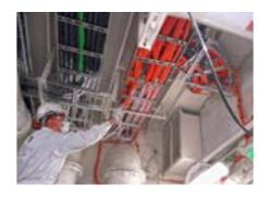
During a fire, the coating expands and protects the cables from fire damage and also prevents the fire from spreading via the cable trays. FS coated cables function during a fire, and if the fire is ceased within a reasonable time, there will be no need for cable replacement.
