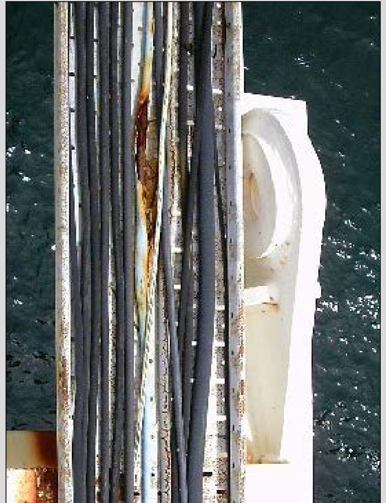
UV7 About to expose inner core
