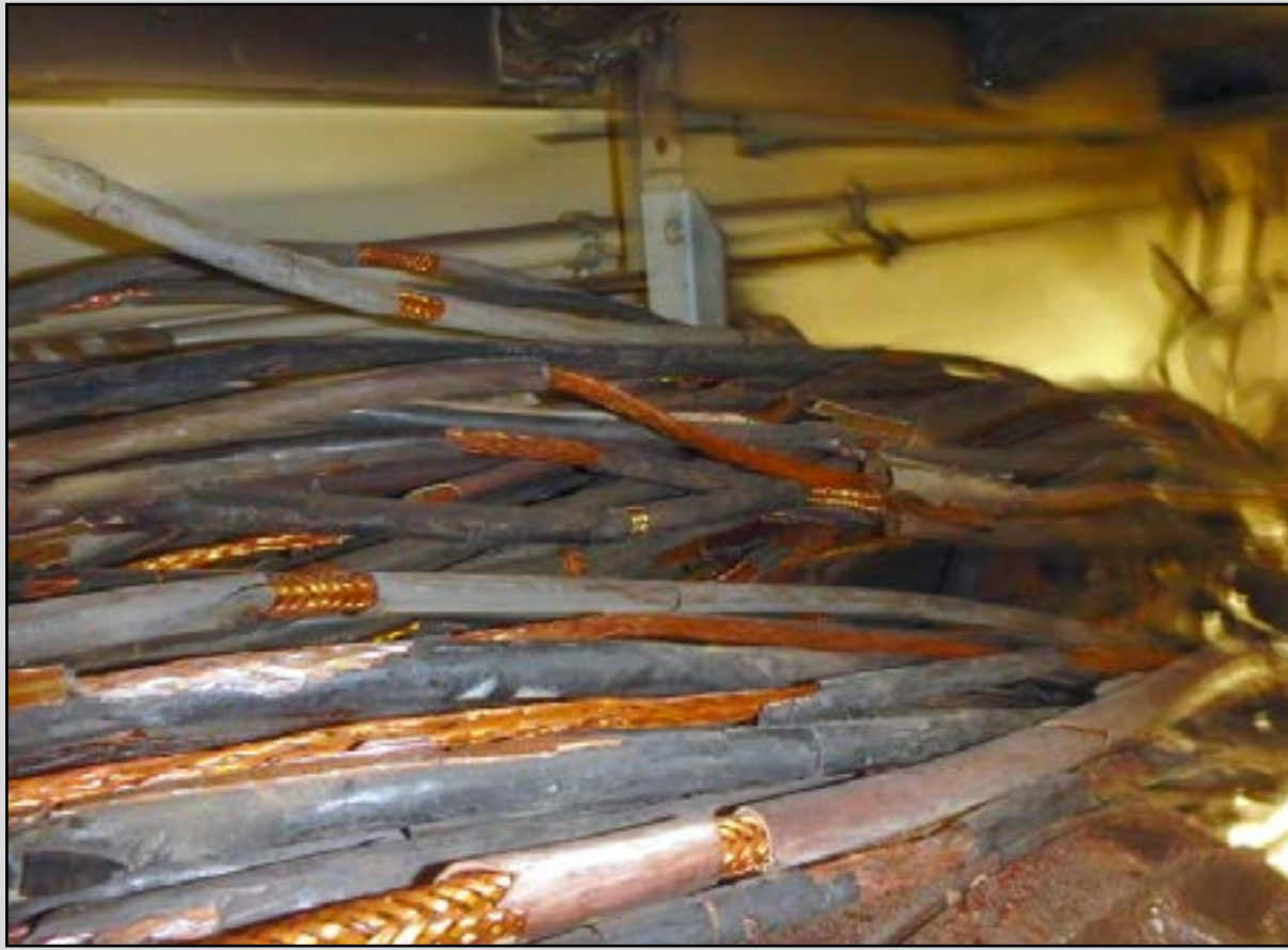
Cables that have been affected by fire but are still capable of operation. FS17 tape repair and coating with FS5.
