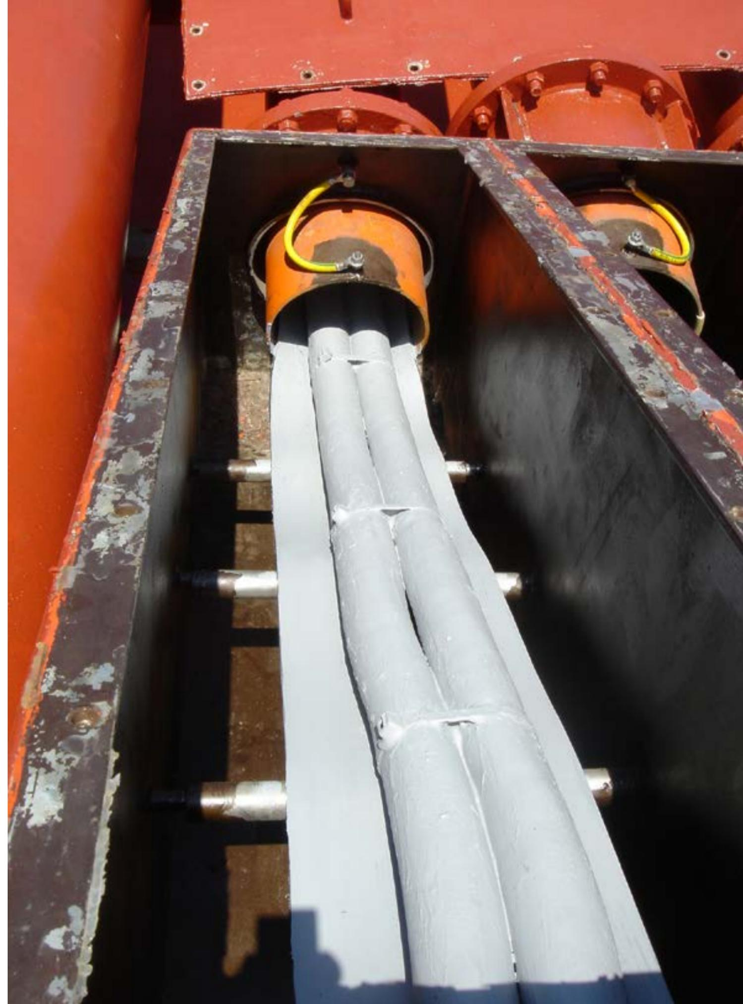
FS repair system fully repair chafing damages and prevent further chafing to occur in the future.
