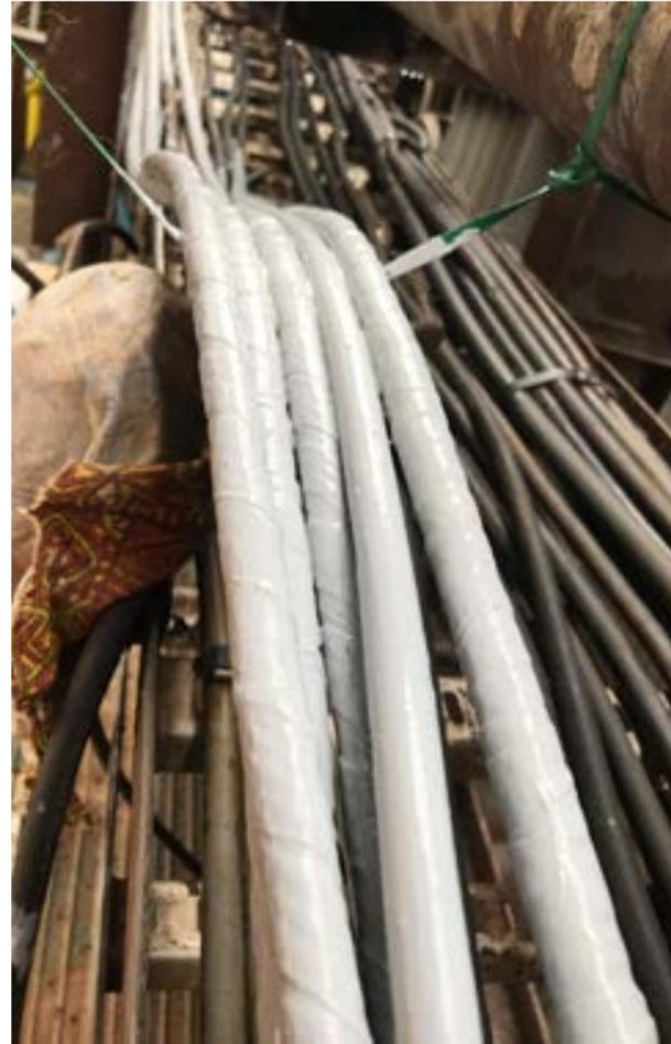
**Oil, drilling mud and hydraulic fluid softens and damages cable sheaths**
