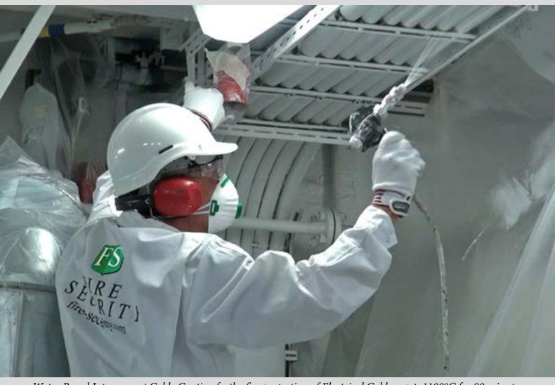
$Water\ Based\ In tumescent\ Cable\ Coating\ for the\ fire\ protection\ of\ Electrical\ Cables\ up\ to 1100^{o}C\ for\ 90\ minutes.$
