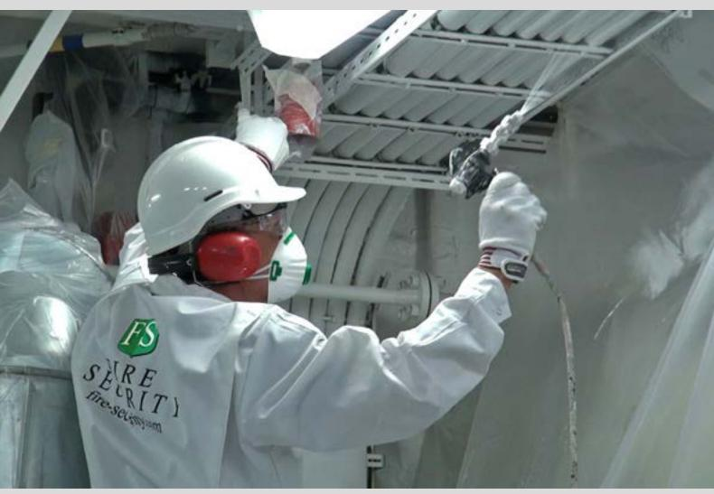
Water Based Ablative FM Approved Cable Coating for the fire protection of electrical cables up to 90 minutes.
