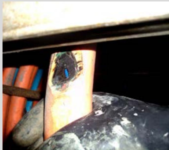
FS Coating brings back and upgrades insulation properties, FS offers to repair cables where the outer sheath is damaged.
