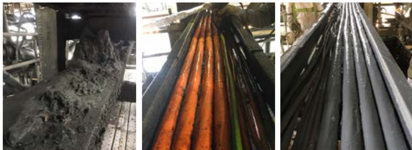
Using warranty backed applications only, FS repairs and upgrades damaged cables.
